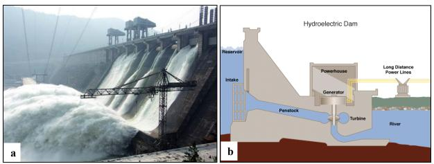
**Figure 5.10.** a) Hydroelectric facility (credit: Denis Belevich, Wikimedia Commons); b) An illustration showing how water is funneled through a portion of the dam to rotate turbines and generate electricity. (Image from Wikimedia, public domain).
